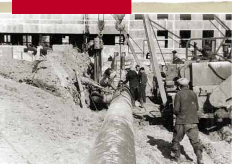
Vyktulskoe field. Above: the drilling foreman Glinski. Below: laying the underground communications to Pumping/ Heating Station of the head facilities © Gazprom, 2015
