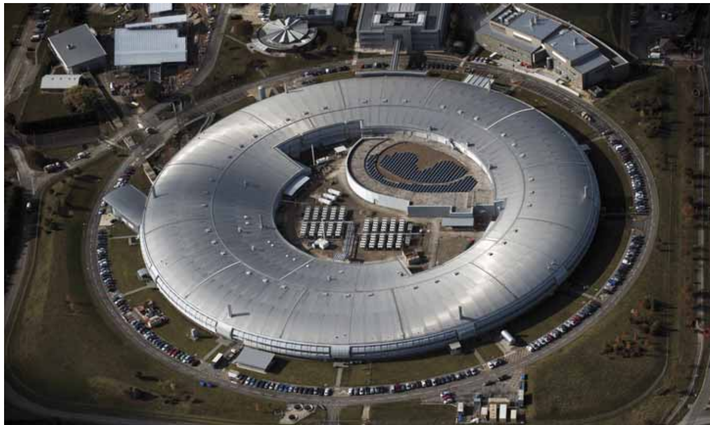
The accelerator at Diamond Light Source generates synchrotron radiation in the range from infrared to X-ray wavelengths. The storage ring is a 24-period structure with a 562-m circumference; the electron beam energy is 3 GeV. The construction costs of Diamond were £260 million; the annual budget, including research costs and operating expenses, is £50 million. Today, there are 25 beamlines of different specialization (right); eight more are under development. Courtesy of Diamond Light Source LTD
